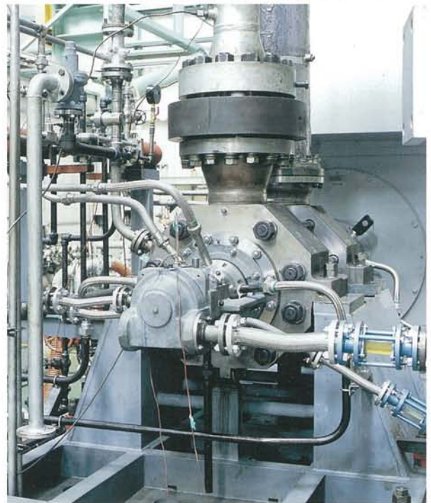
Segmental ring-section casing boiler feed pump 3,018ft-2,100 U.S.gpm-2,980min -1 -2,050HP Fujairah Power Plant(Abu Dhabi), 660MW
