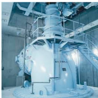
Dewatering pump with adjustable vane (Size:2400mm, Driver:1103kW)
